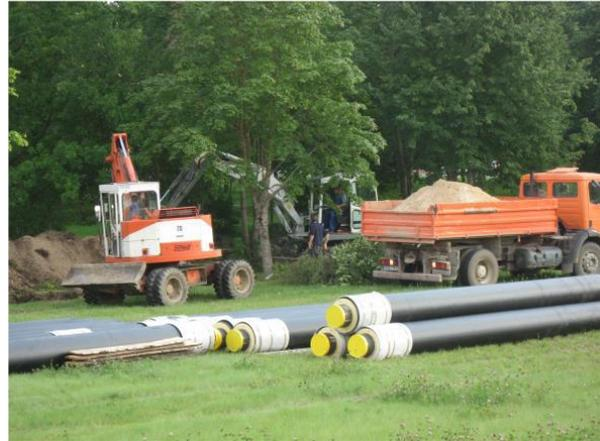
Figure 13 New cased underground pipelines
