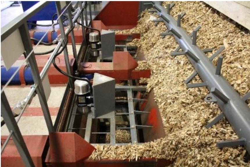
**Figure 9 Feed-in system of a woodchip boiler**
